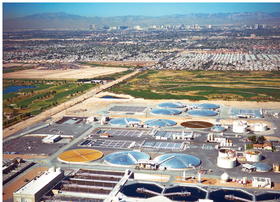
Figure 4.18 Pure piped water replacing individual or neighborhood wells, and sewers and waste treatment plants instead of privies, became increasingly common in urban Europe and North America during the 19th century. Their modern successors, such as the Las Vegas, Nevada, treatment plant shown here, helped complete the epidemiologic transition in developed countries. Lynn Betts, USDA, Natural Resources Conservation Center
